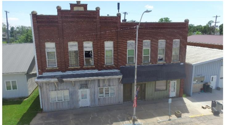
Although originally the plan was to deconstruct the buildings and salvage/recycle as much material as possible, the site has been deemed structurally unsafe to enter due to ongoing decay/water intrusion. Therefore, the 211 and 213 E Broadway St buildings will be fully demolished through RACM demolition and all building materials will be disposed of properly.
