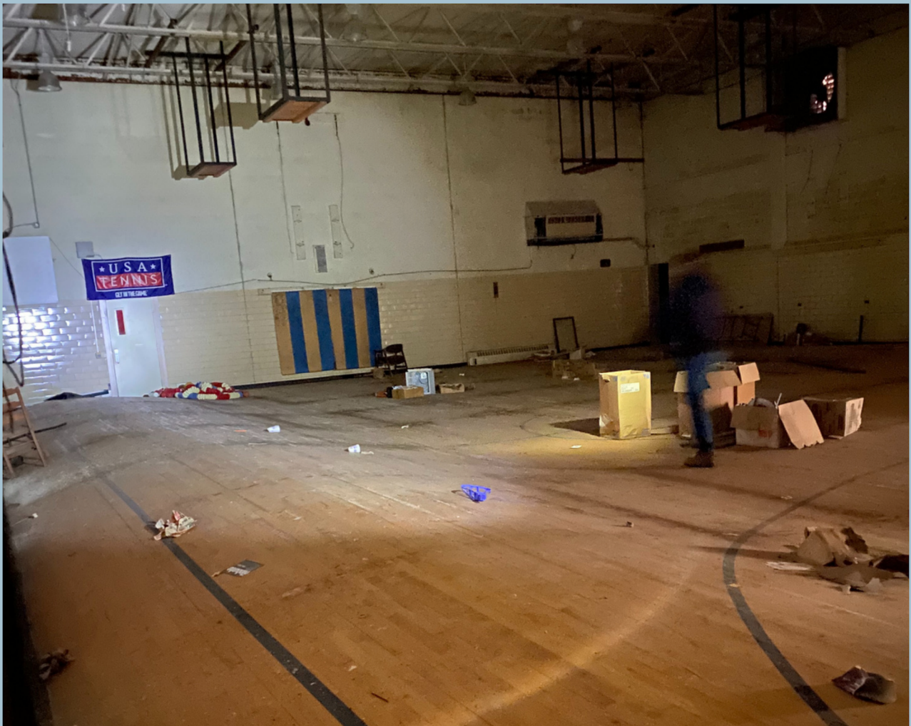
Pictured: YMCA Gym Floor Damaged Due to Water
