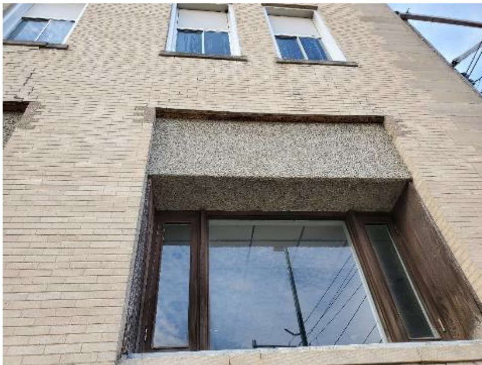
Photo 16: View of 1905 Bldg. exterior window caulk around window frames, gray (HA-15).
