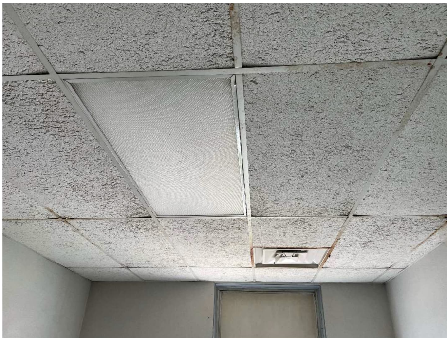
Photo 14: View of moisture-impacted ceiling tiles and ruset ceiling tile grid inside Unit 201 on second floor
