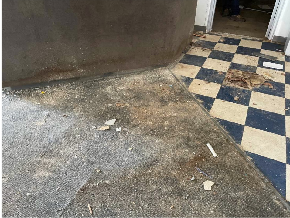
Photo 9: View of water stained flooring on first floor near Room 3/behind the counter
