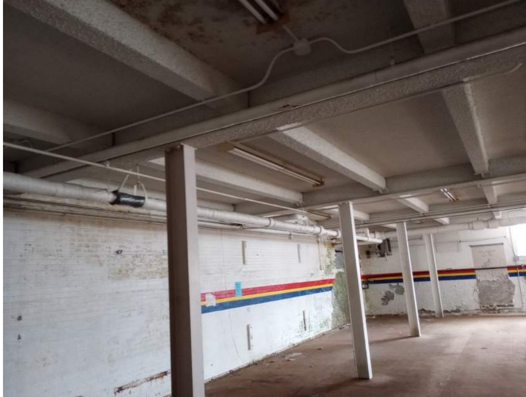
Wood and Steel framed Construction in Basement Under Lobby
