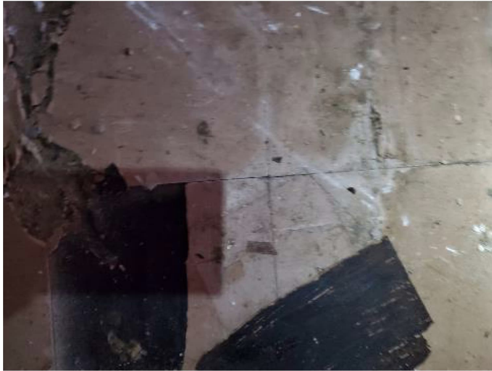
Photo 11: View of 1905 Bldg. 2 nd floor, near the restrooms, 9" x 9" floor tile & mastic (PC8-22).
