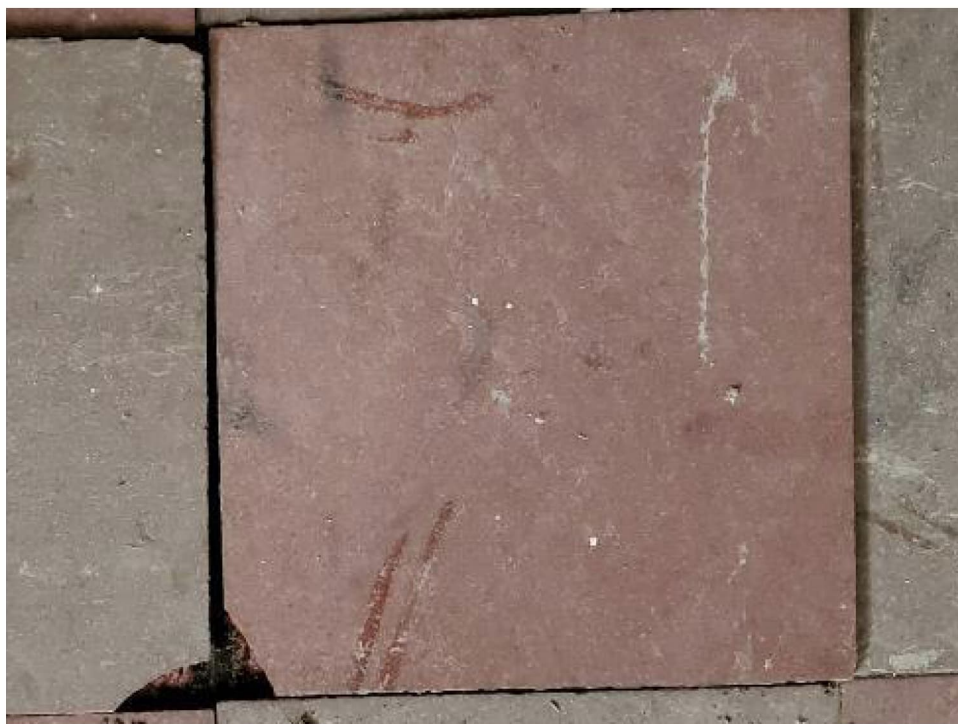
Photo 8: View of 1905 Bldg. basement, 9" x 9" floor tile and mastic, southeast room, corner (PC5-13).
