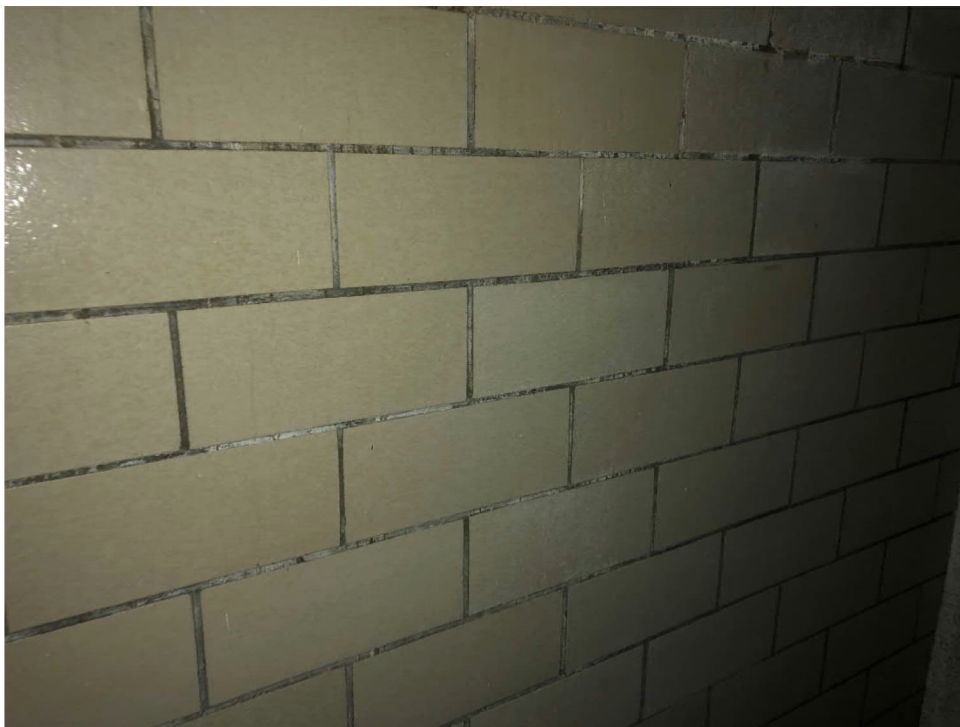
Photo 2: View of LBP on glazed ceramic block in locker rooms
