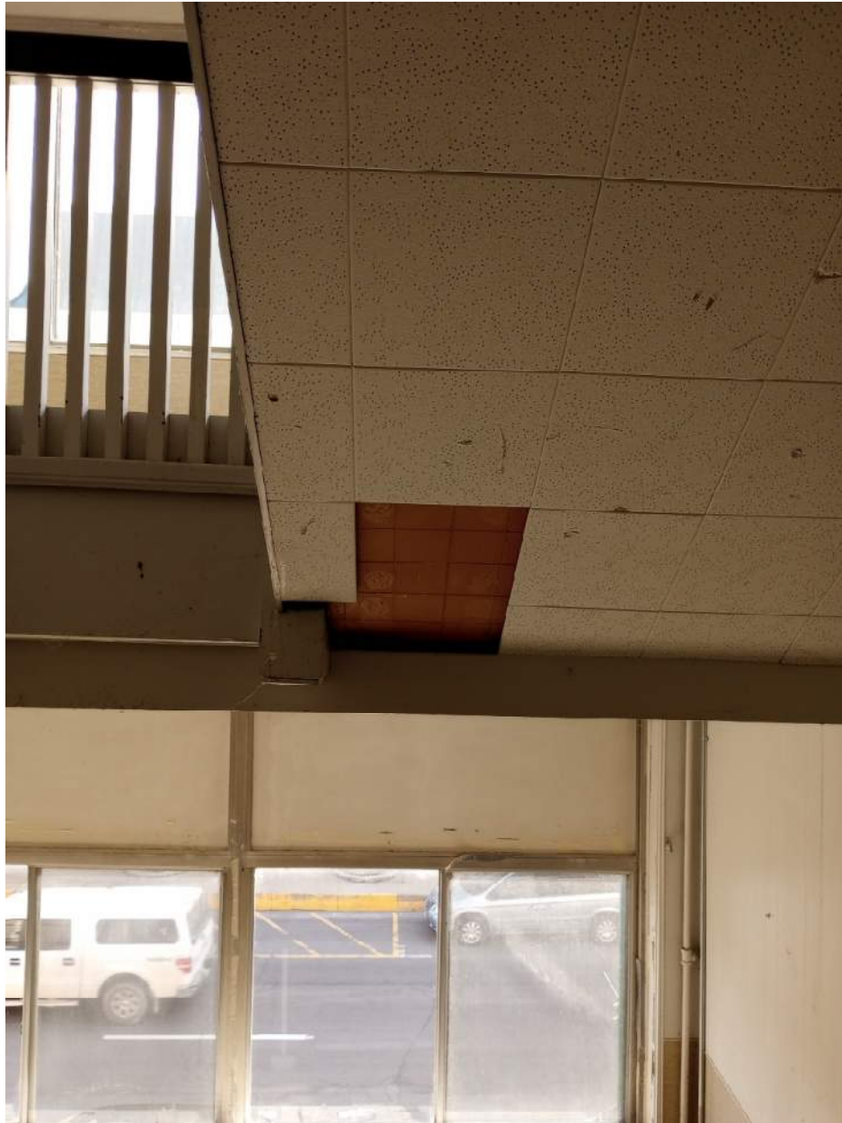
Non Structural Tile – Potential Asbestos Abatement
