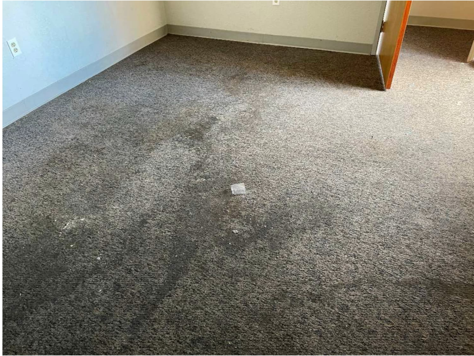
Photo 19: View of water damaged flooring in Unit 318 on third floor
