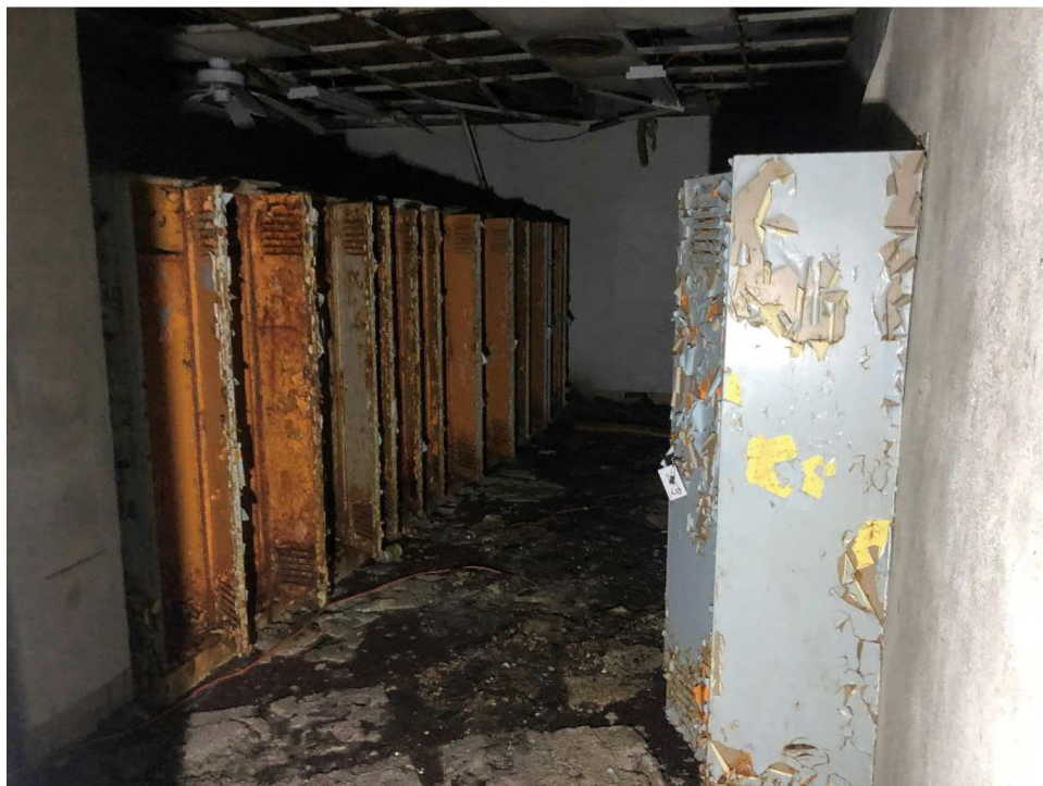
Photo 6: View of LBP on lockers
