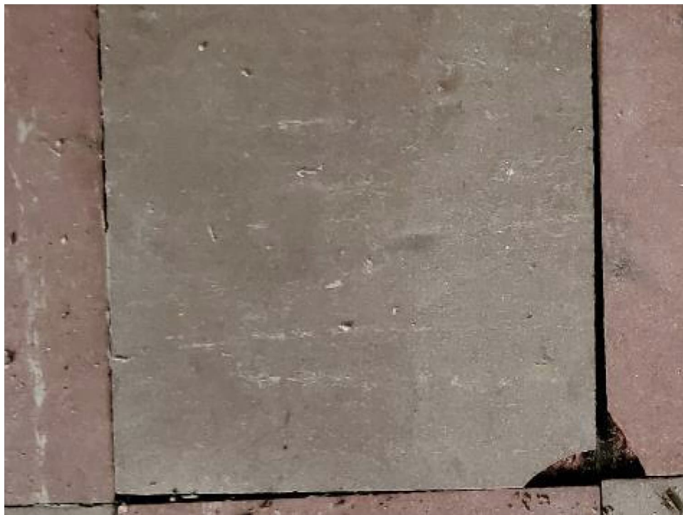
Photo 14: View of 1905 Bldg. basement, 9" x 9" floor tile & mastic, southeast room, corner (PC14-40).
