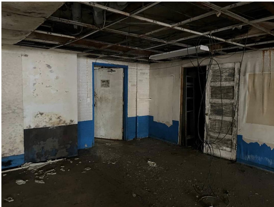
Photo 22: View of water damage and suspect microbial growth in northwest portion of basement
