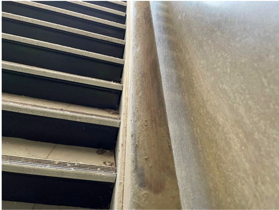
Photo 13: View of handrail leading from first floor to second floor with water damage and suspect microbial growth
