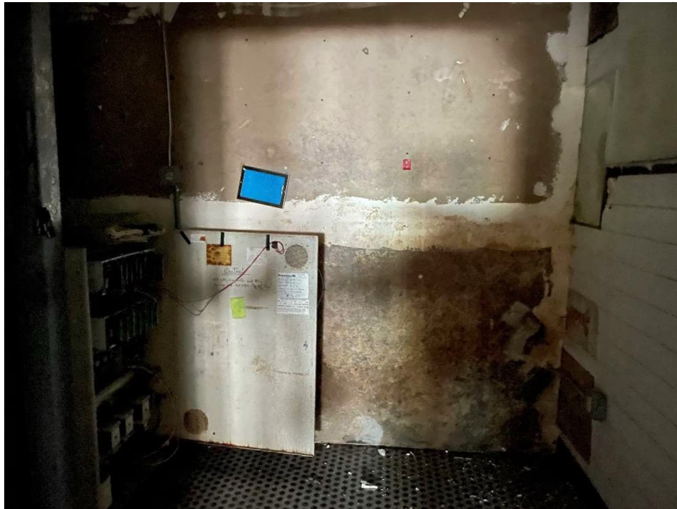
Photo 21: View of significant water damage in Room B8 in the basement
