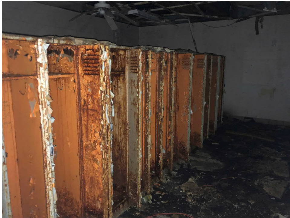
Photo 5: View of LBP on lockers
