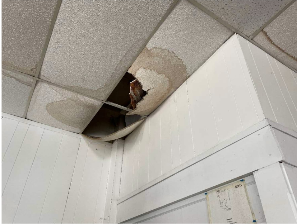
Photo 17: View of water damaged ceiling tiles at southwest corner of Room 11 on second floor
