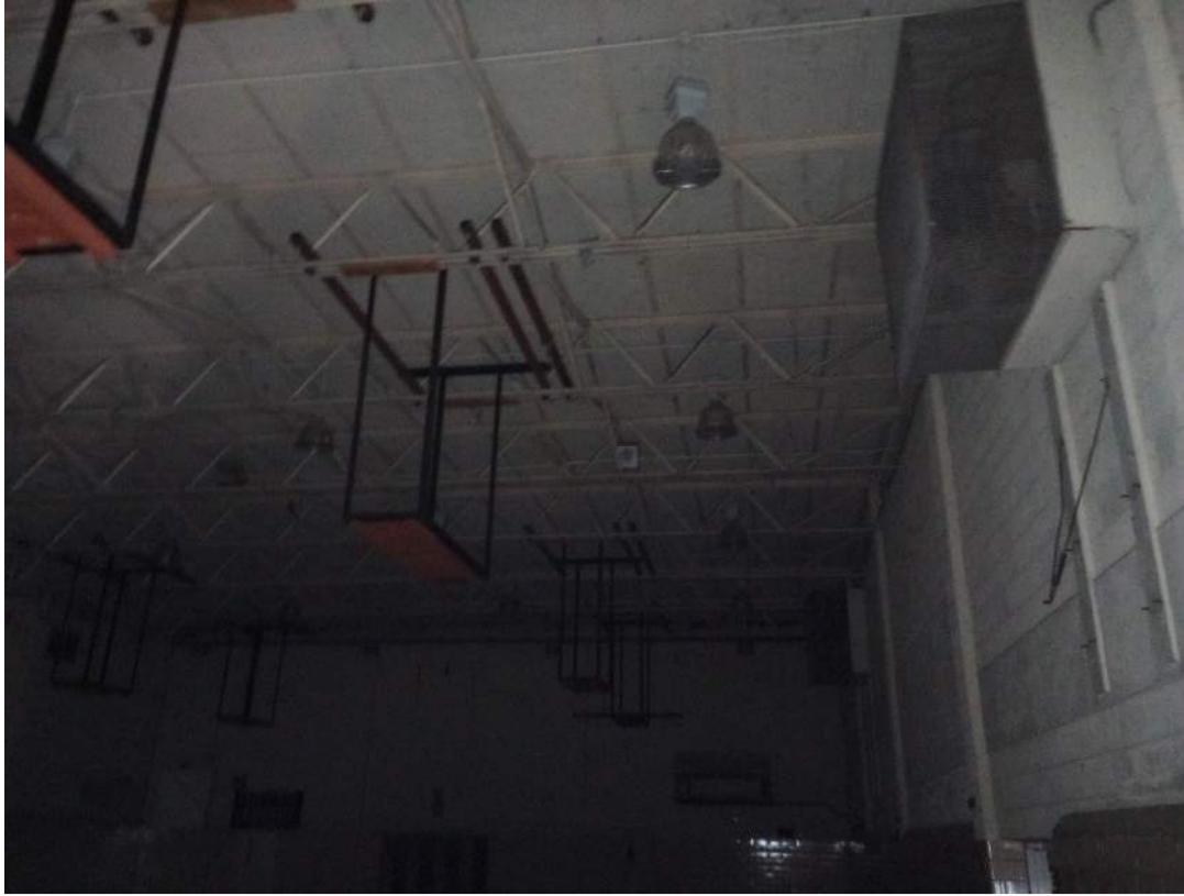
Steel Roof Framing on Second Story of Building B2
