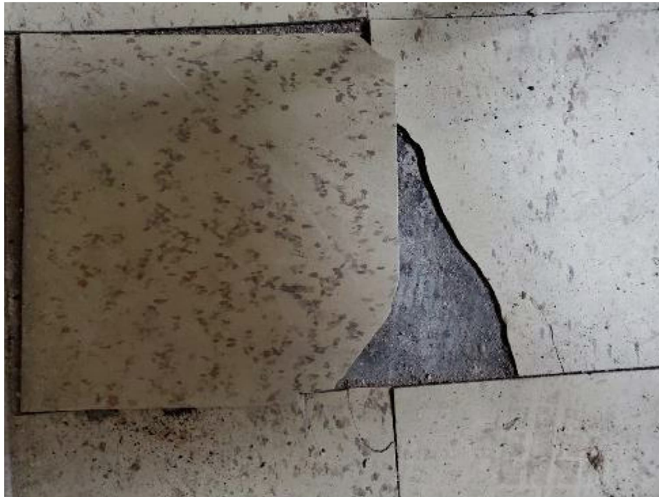
Photo 9: View of 1905 Bldg. 1 st floor, southeast room, 9" x 9" floor tile, (PC6-16).
