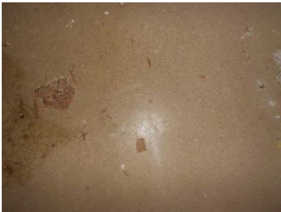
Photo 2: View of 1905 Bldg. 2 nd floor, 9" x 9" floor tile, south restroom, beneath vinyl flooring (NC-04).
