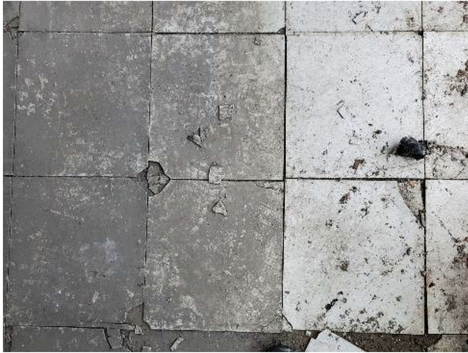
Photo 13: View of Bldg. 1961 1 st floor, main lobby, 12" x 12" floor tile & mastic (PC13-37).
