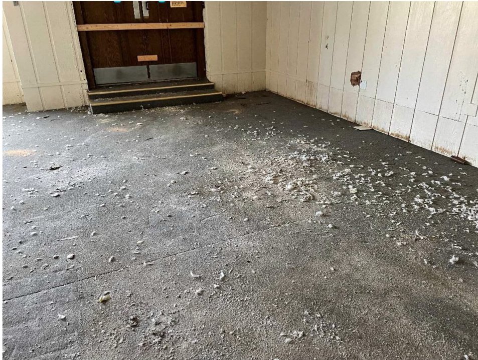
Photo 11: View near southeast corner of Room 5 on first floor with water damaged flooring and water staining on wood paneling
