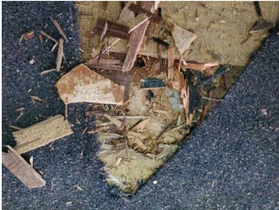
Photo 3: View of 1905 Bldg. 1st floor, 9" x 9" floor tile in main lobby, beneath underlayment (NC-16).
