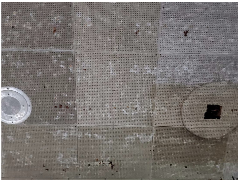
Photo 18: View of 1961 Bldg. 2" x 2" cement board pegboard panels, gray (HA-22).
