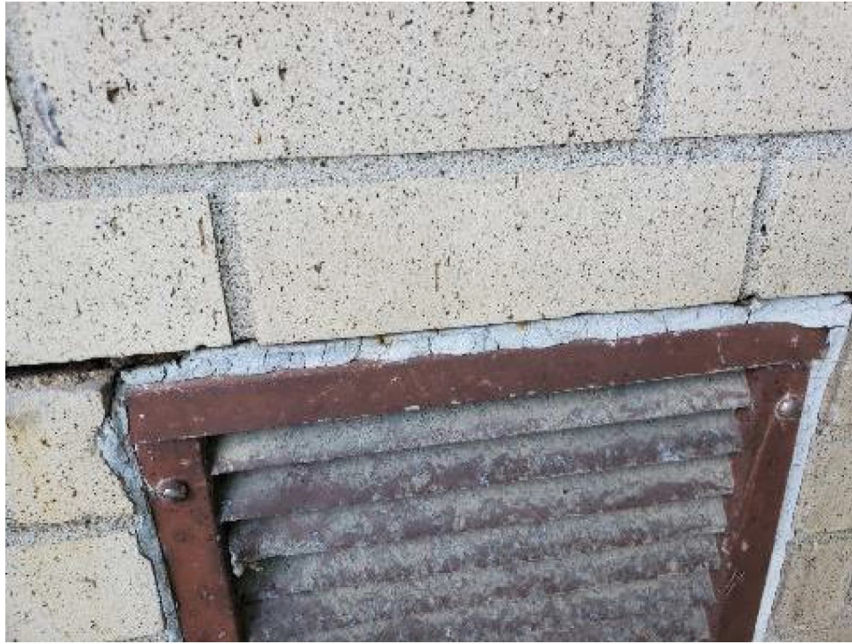
Photo 16: View of 1961 Bldg. exterior north wall, gray caulk on building exhaust (HA-15).
