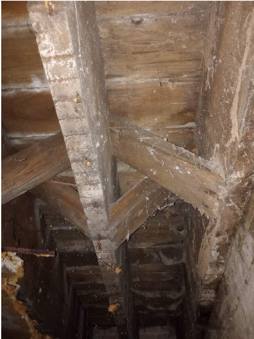
Uncompromised Wood Structure in the Floor Cavity of Building A
