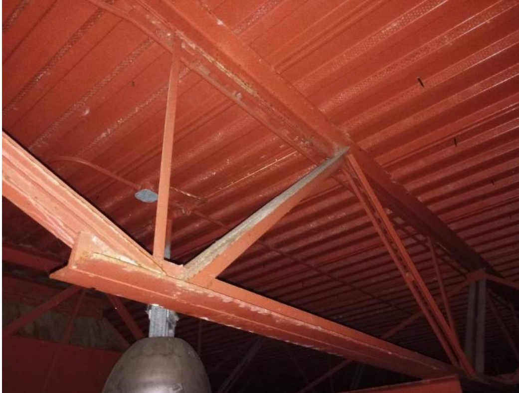
Painted Steel Roof Joists at Gym Area
