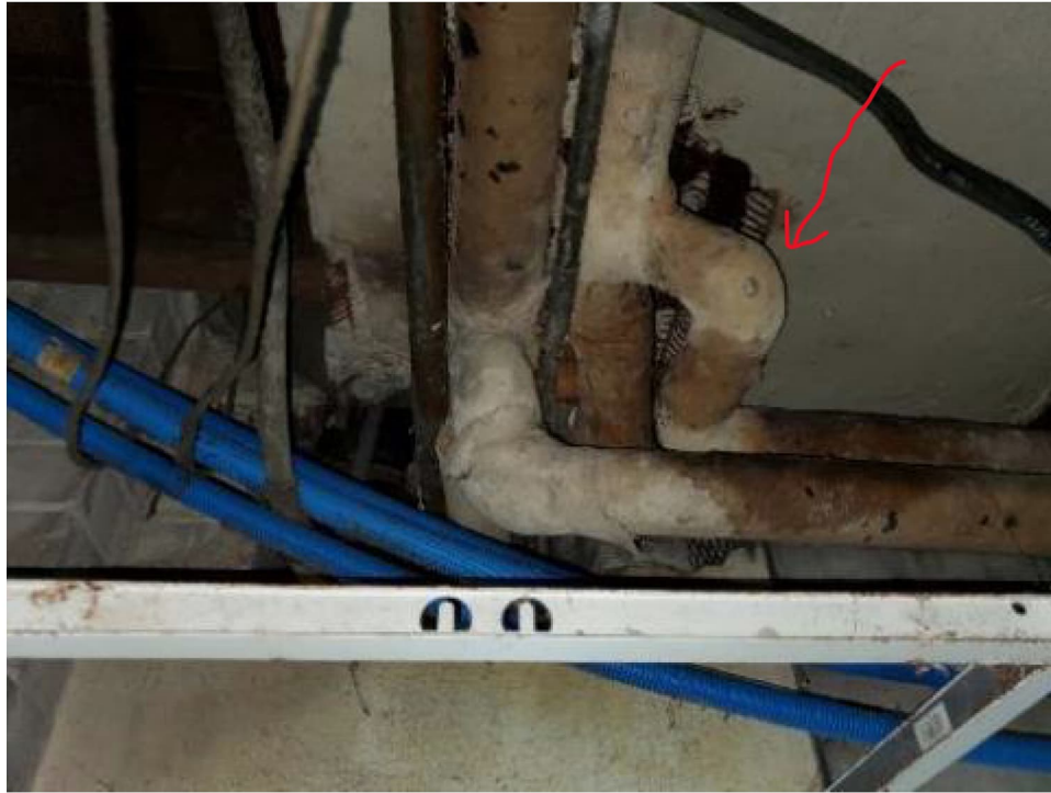
Photo 5: View of 1905 Bldg. basement, mudded joint fitting with canvas wrap (PC2-04).
