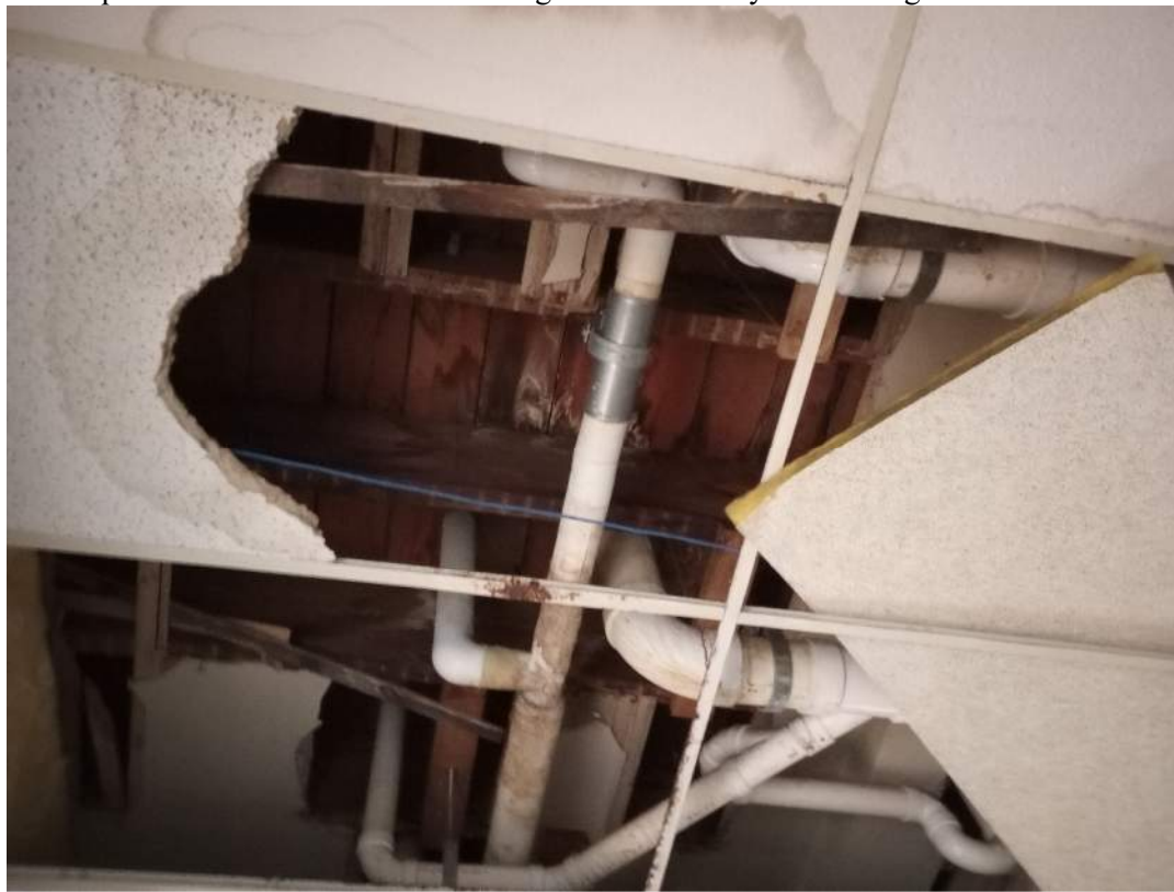
Uncompromised Wood and Steel Framing in Second Story of Building A
