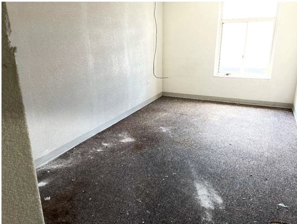
Photo 18 View of water damaged flooring in Unit 323 on third floor
