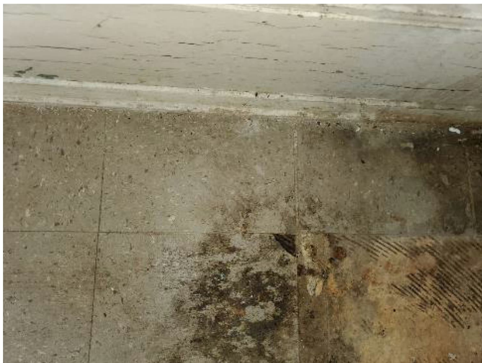
Photo 10: View of 1905 Bldg. 1 st floor, storage room, 9" x 9" floor tile (PC7-19).
