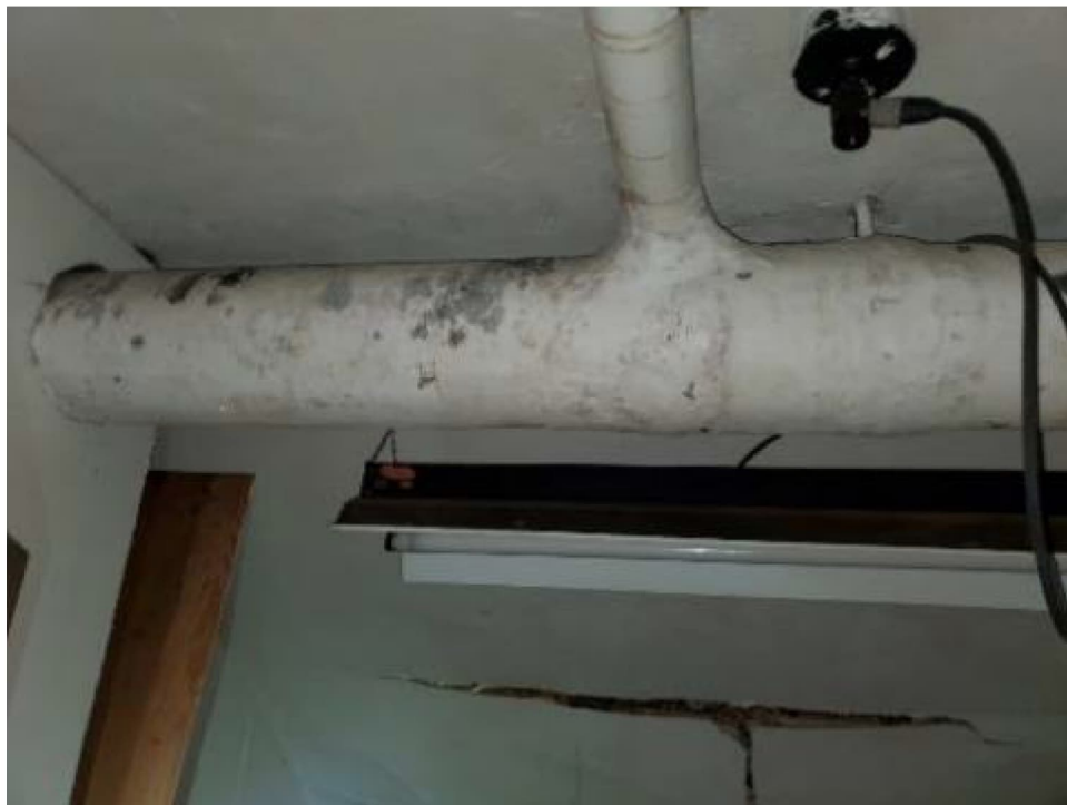
Photo 4: View of 1905 Bldg. Mag. Pipe insulation, basement landing of east stairwell (PC1-01).
