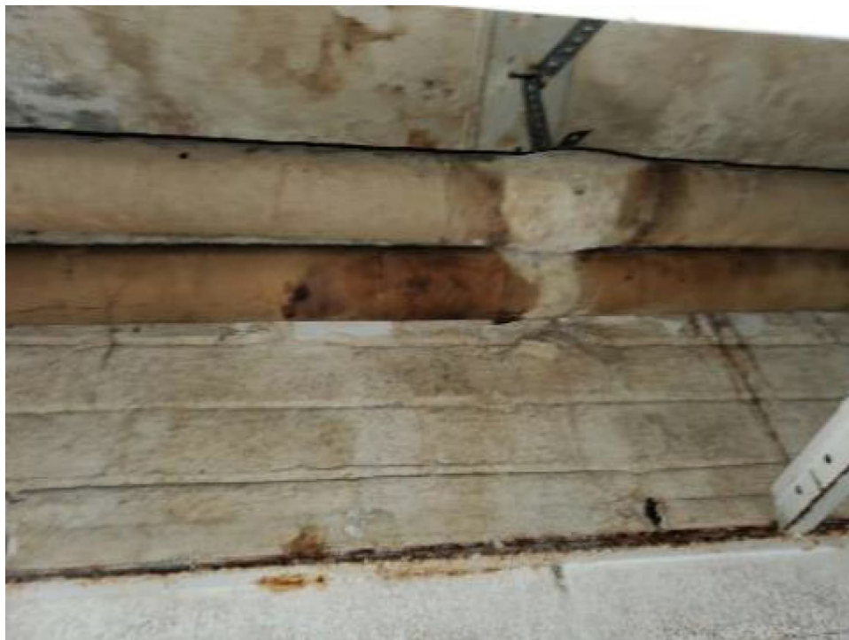
Photo 6: View of 1905 Bldg. basement, mudded joint fitting w/ canvas wrap on fiberglass pipe (PC3-07).
