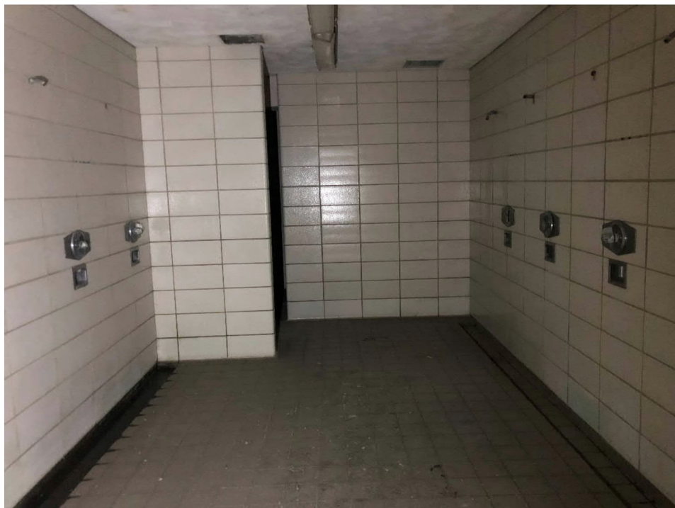
Photo 4: View of LBP on glazed ceramic block in locker rooms
