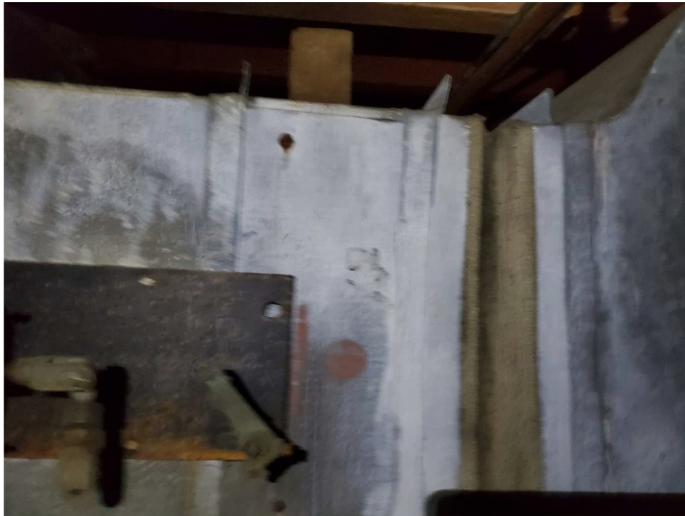
Photo 17: View of 1961 mezzanine mechanical room vibration cloth, white (HA-17).
