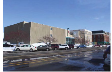
Front of Property
