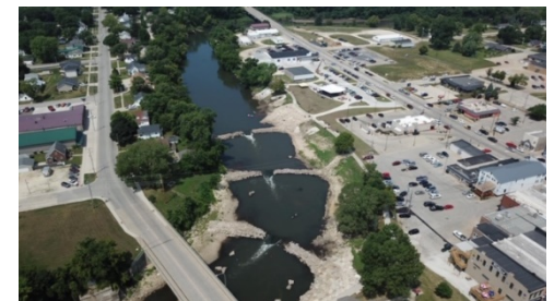
Aerial View of Whitewater park after completion
