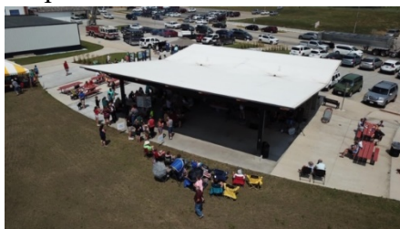
Picnic pavilion and restrooms after redevelopment
