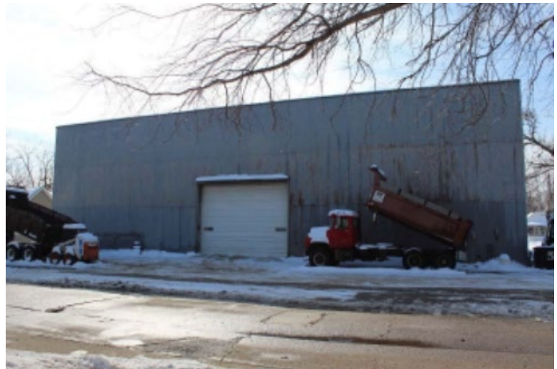
Street view - Front of Warehouse
