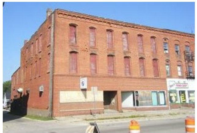
1006 S 4 th St adjacent to property
