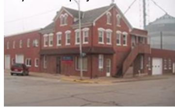
Dyersville- project site
